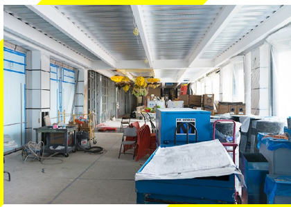
The exposed corrugated steel ceiling in the Commons.
